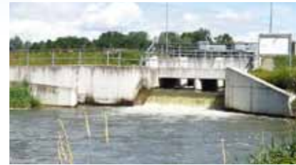
▲ Sluice gate to Ottheinrichbach with fish way (left)
